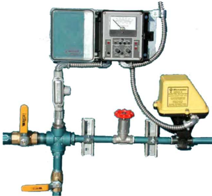
Example of an automated , conductivity-based blowdown flow control set up
